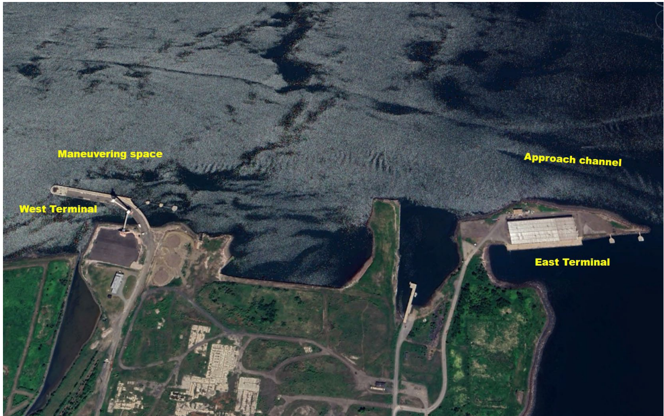
Figure 1 : Approach channel to the West terminal.
